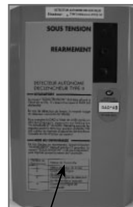
Smoke detecting station
